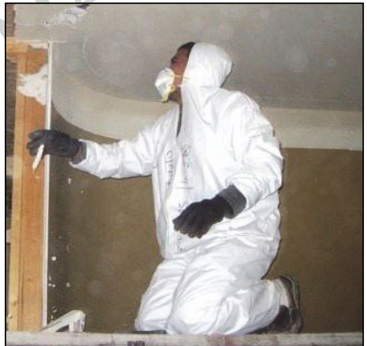
Photo 5: During demolition, workers should wear a minimum of goggles, gloves, and an N-95 respirator for protective gear. The worker above lacks eye protection and is improperly wearing his respirator straps.
