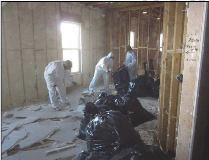
Photo 6: CDW can be disposed of as general demolition waste but must never be recycled.
